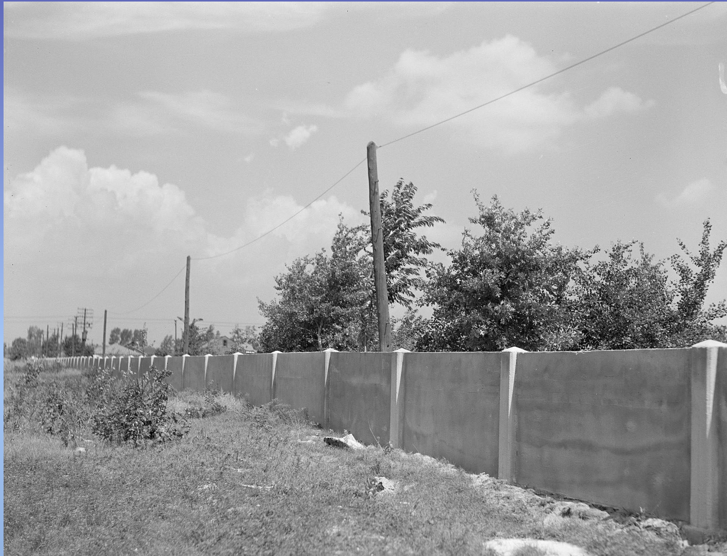
Eight-mile (Birwood) Wall, Detroit (1941)
