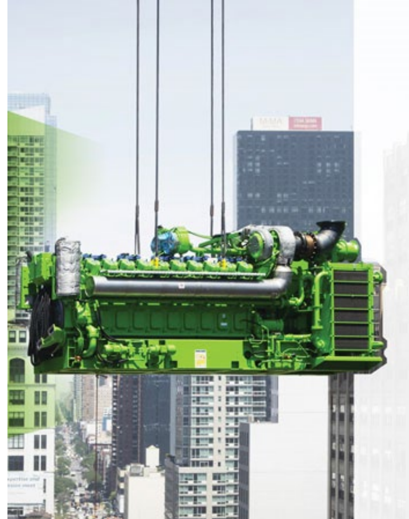
CHP unit being lowered by crane into Hudson Yards
