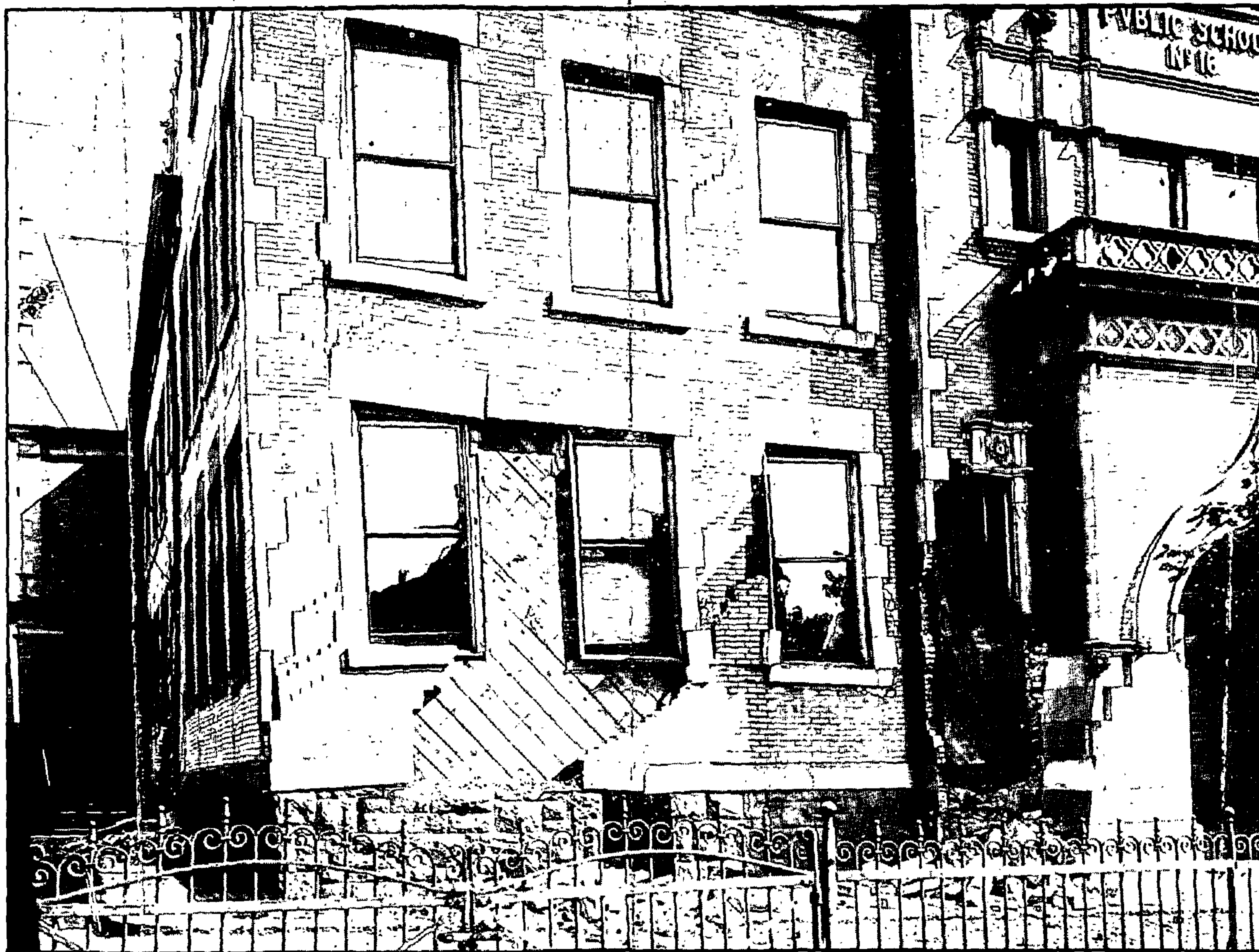
Wrecked by a mine cave on August 29, as school was to open a week later. Had this occurred a few days later, when 500 pupils were assembled for classes, a panic would have resulted. The total damage of this cave is estimated at $50,000.
