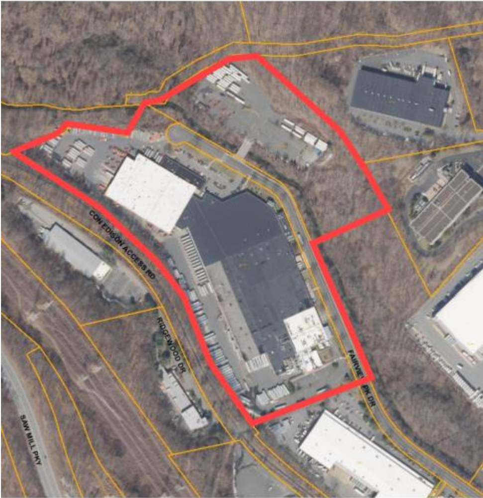
Coca-Cola 440,000 sq. ft. facility 22-acre site
