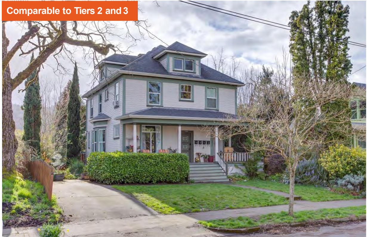
A four-plex on a 5,014 square-foot lot on 9426 N Edison St in Portland, OR.
