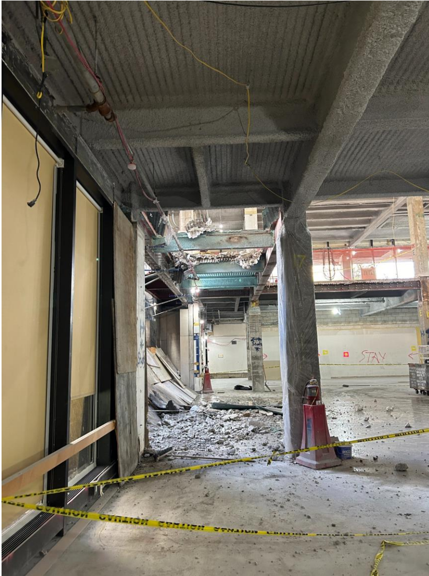
West side courtyard facing structural slab demolition.
