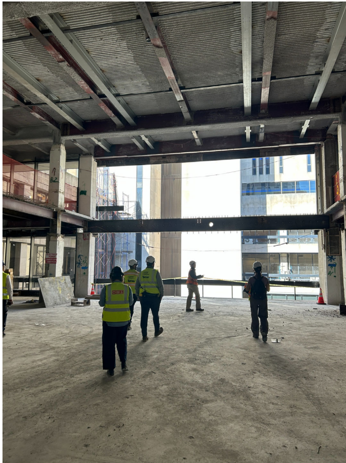
Façade demolition is complete for future Medium Venue.
