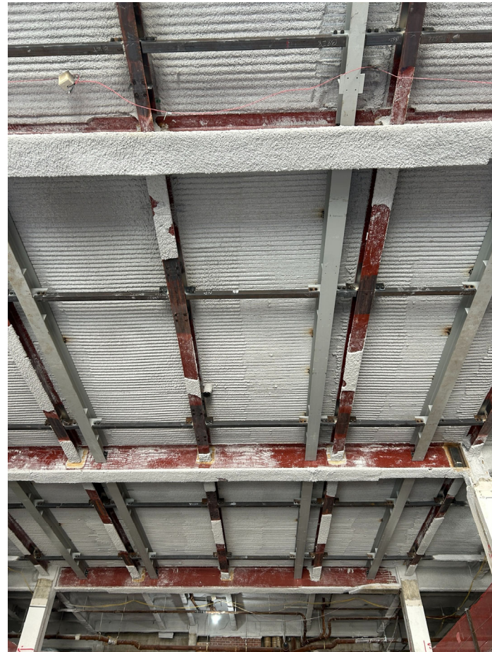
New structural steel installation at Medium Venue.
