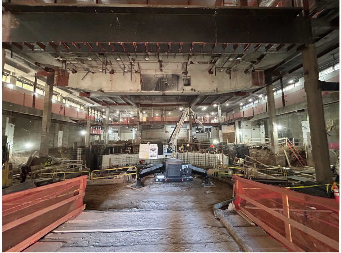
Rebar installation and concrete slab and footing pours ongoing in Large Venue.
