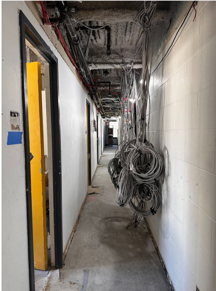
Electrical conduit installation in the Maria's Tower.
