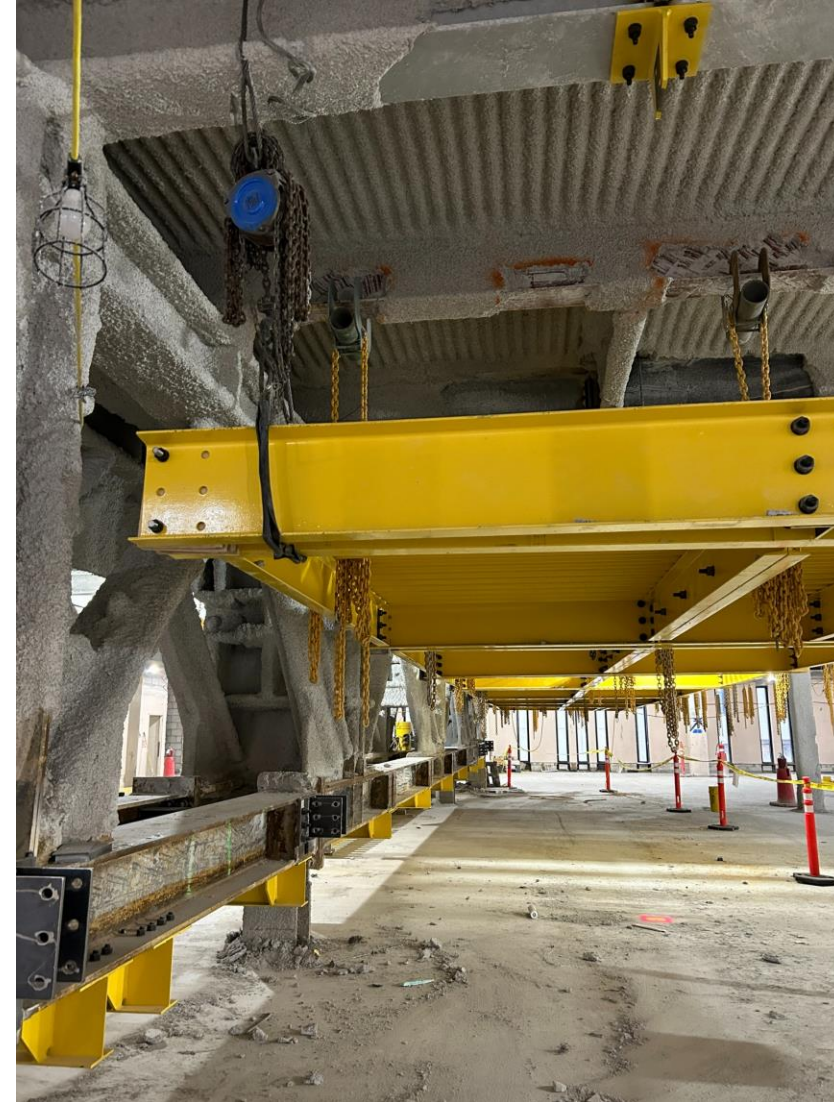
Grid iron being temporarily hung on the 2 nd floor.
