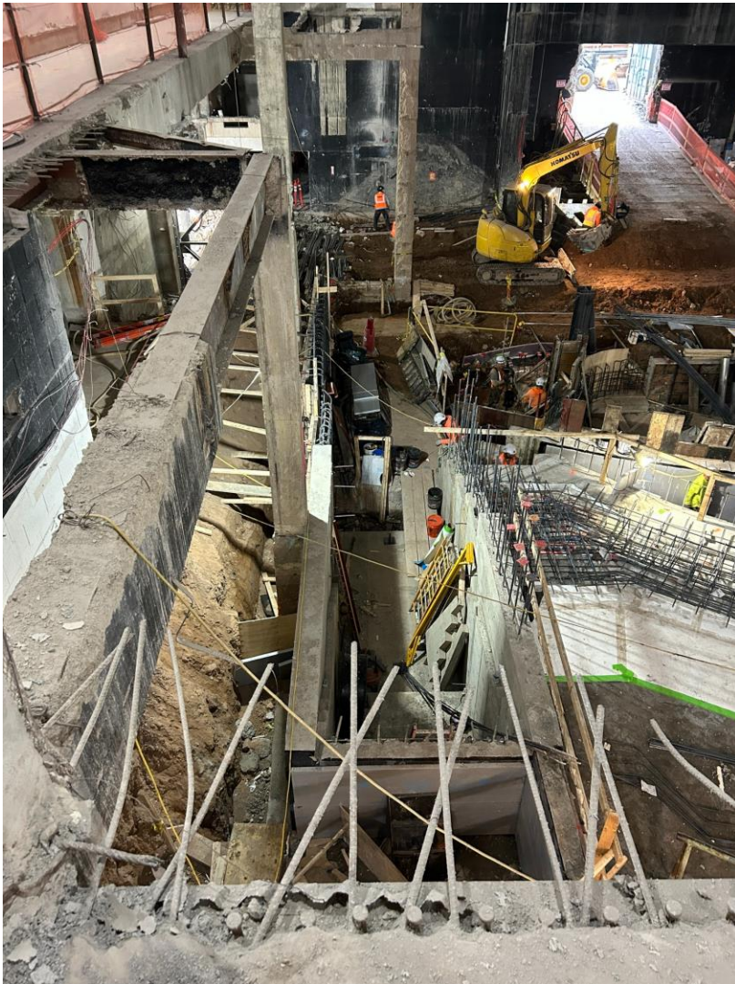
Continued rebar installation in the Large Venue in preparation for the concrete slab on grade.
