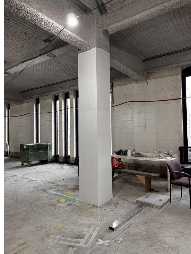
Plaster column finish mockup on the 3 rd Floor.
