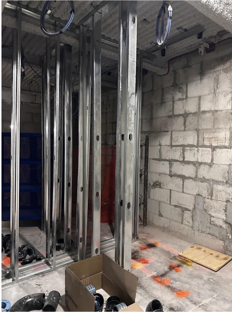
Installation of bathroom framing in Maria's Tower.
