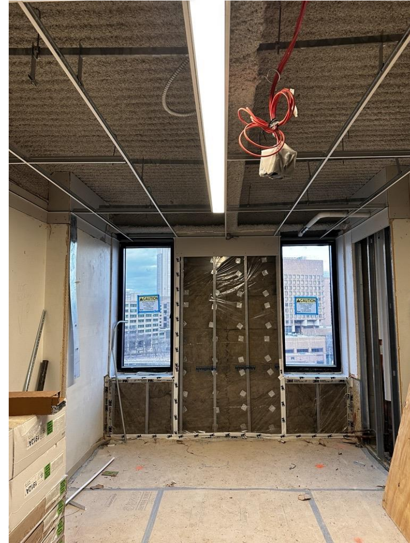
Installation of ceiling grid and lighting in Maria's Tower.
