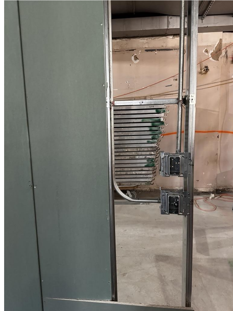
Electrical rough-in work is ongoing throughout.
