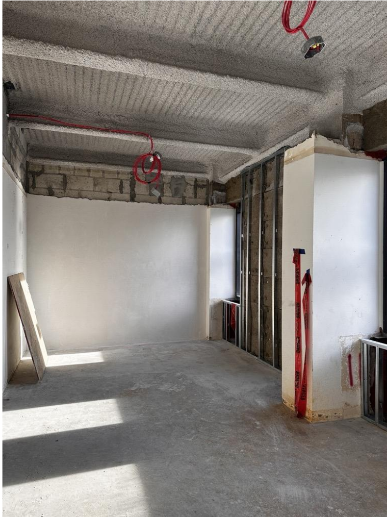
Interior carpentry work is ongoing in Maria's Tower
