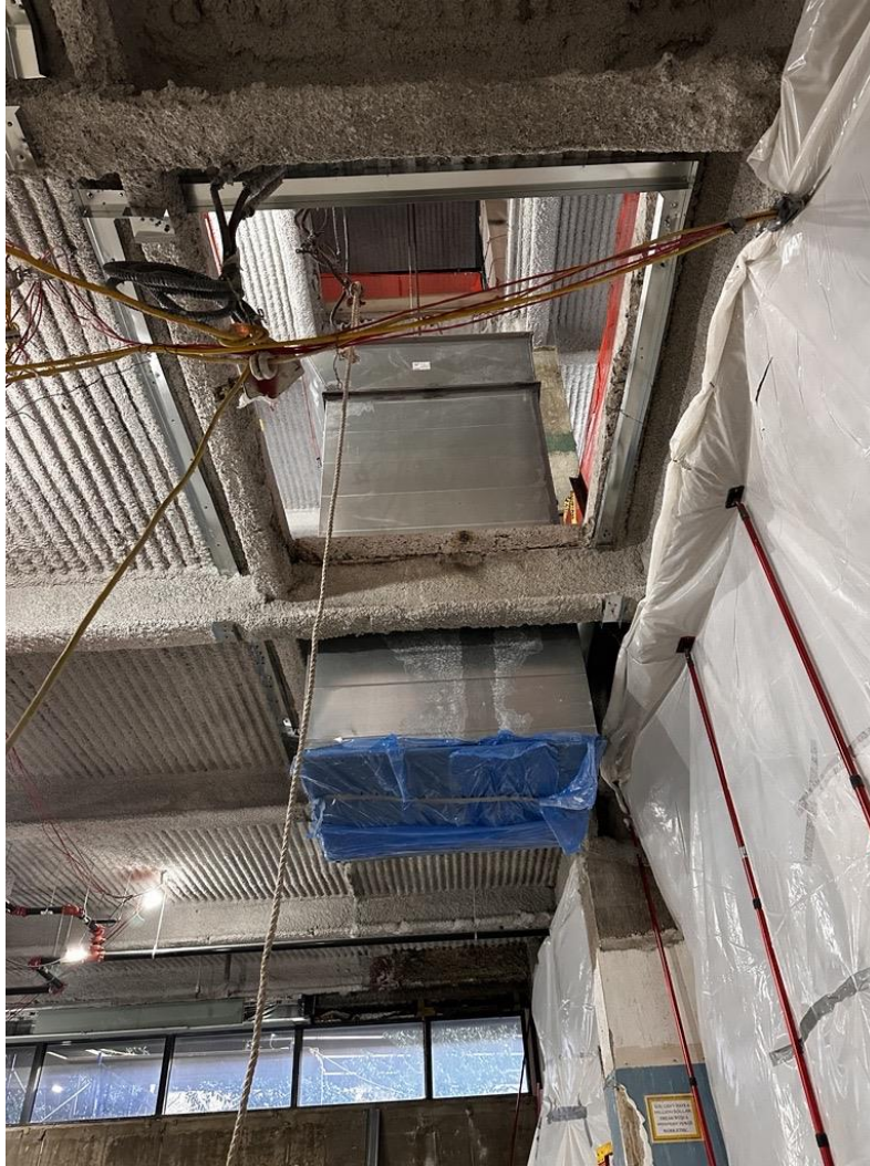
Installation of mechanical risers is ongoing throughout the Podium.
