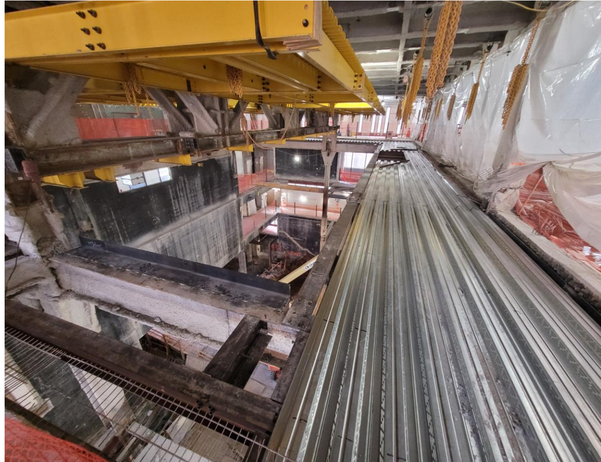
Large Venue decking installation.
