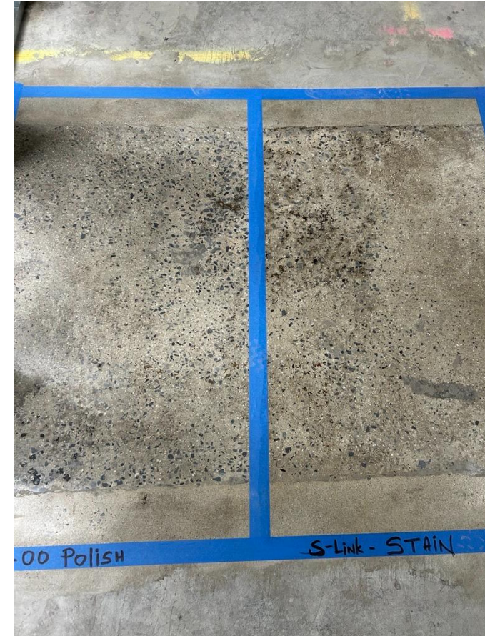
Existing concrete finish mock up for review.
