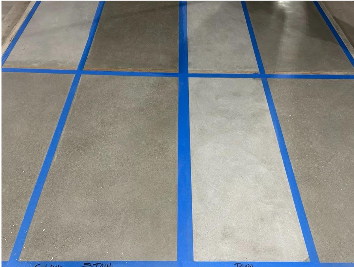
New concrete finish mock-ups on site for the project team review.
