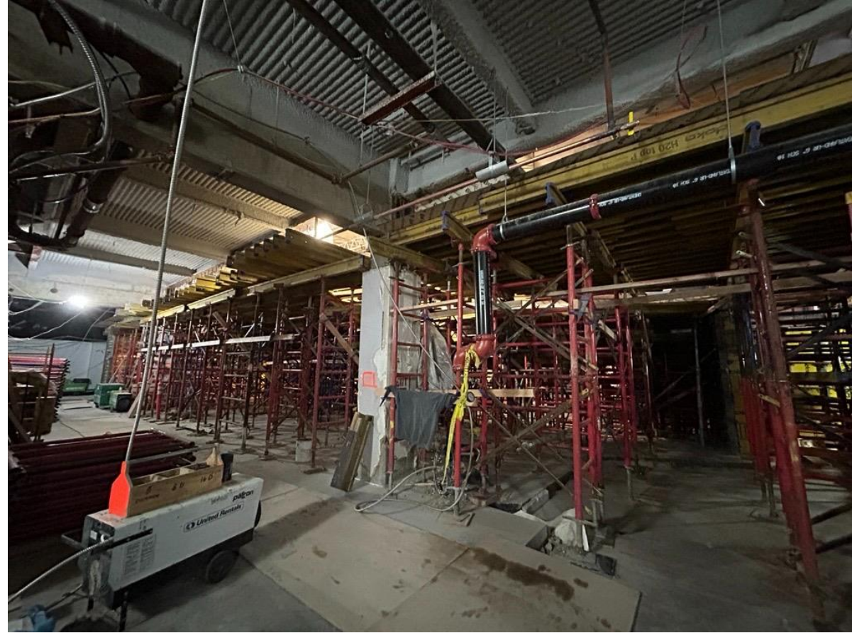
Large Venue audience concrete scope scaffolding and formwork is ongoing.
