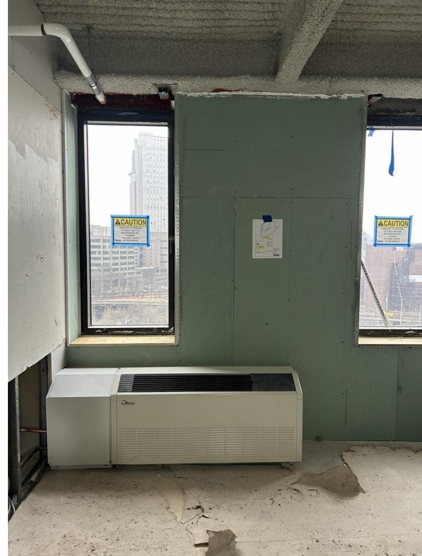
New mechanical unit installation in Maria's Tower.
