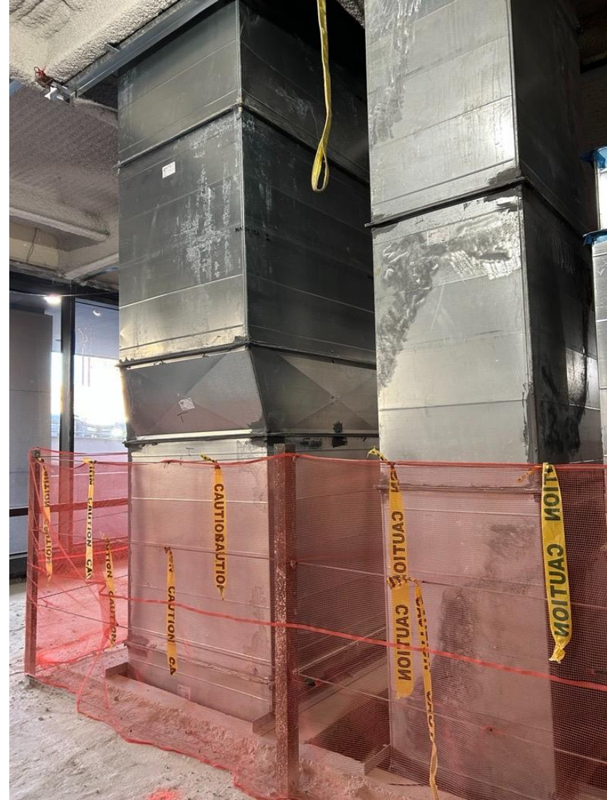
1 st Floor mechanical ductwork installation is ongoing.
