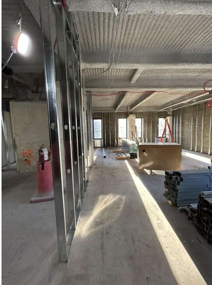
Interior partition installation on the 18 th Floor of Maria's Tower.
