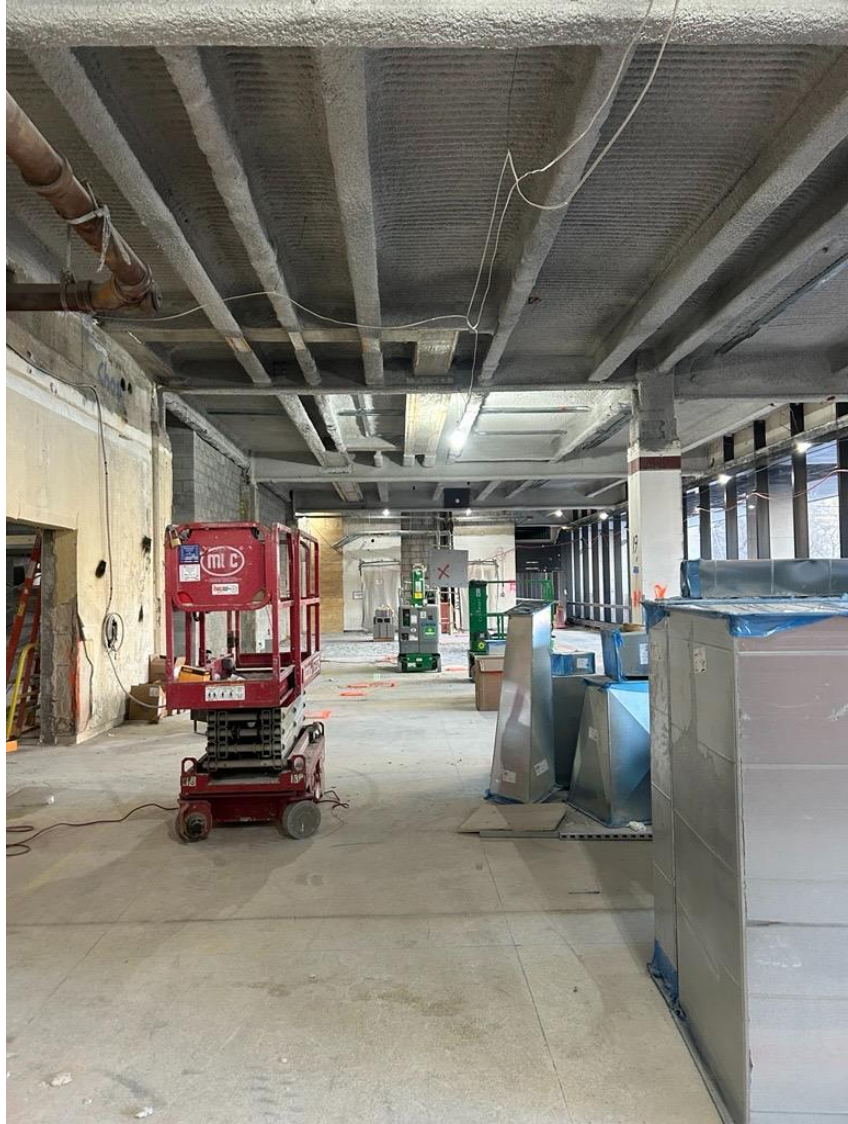
1 st Floor mechanical ductwork installation is ongoing.
