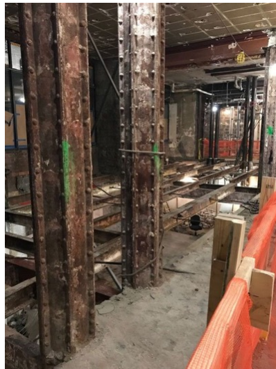
41 Park Row – Stripped column condition
