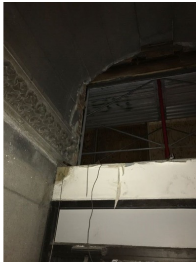
41 Park Row – Uncovered historic arch
