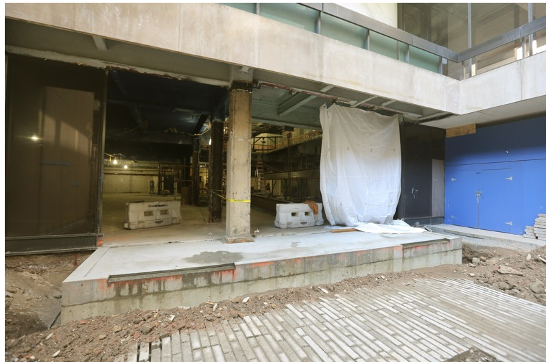
1 Pace Plaza – Foundation and footing work for Lubin Entrance
