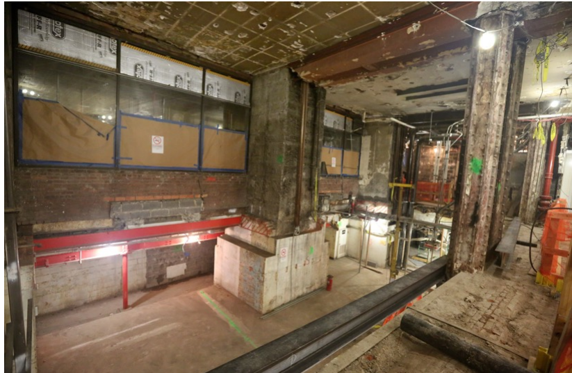
41 Park Row – 1 st floor stair framing
